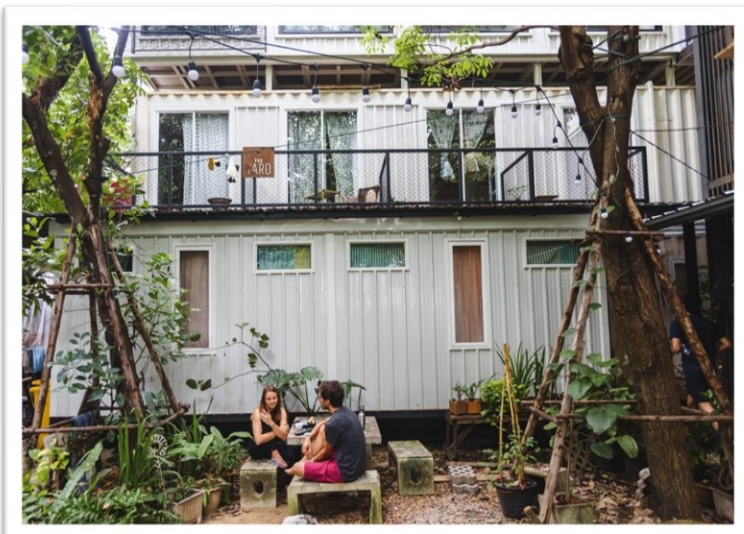
Figure 20: Rooms built from old shipping containers at The Yard Hostel (Hostelworld, s.d.)
